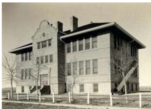
Fire escape tubes
